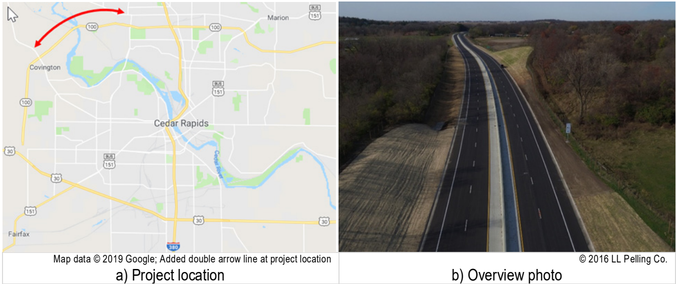
Figure 1. Iowa State Highway 100 project near Cedar Rapids.
