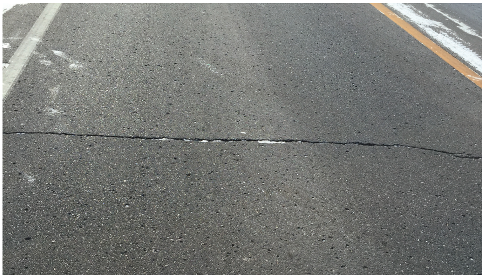
Figure 11. Thermal cracking
