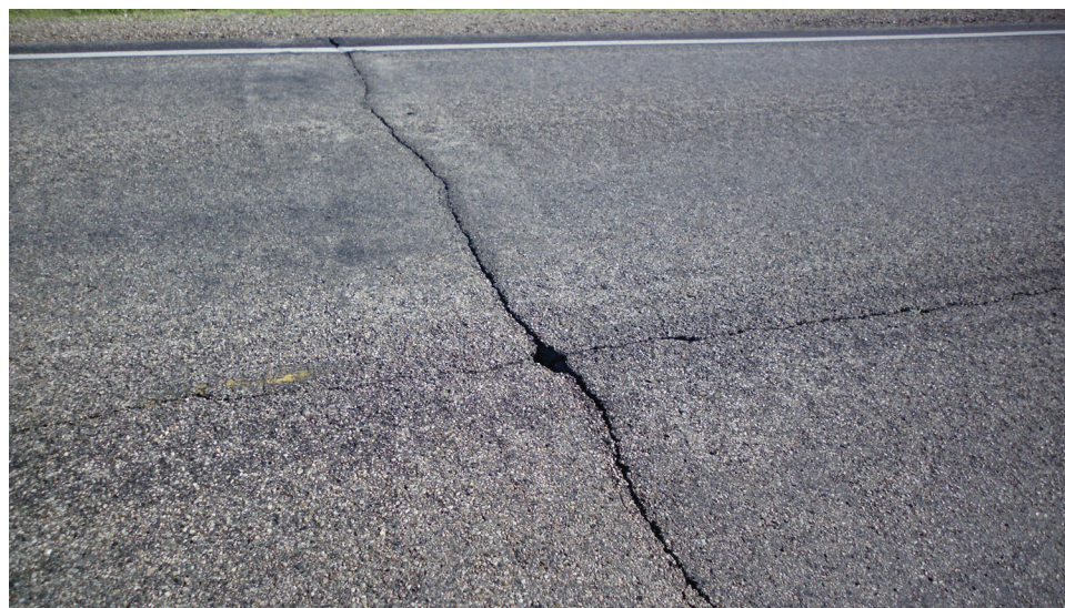
Figure 13. Transverse crack with adjacent snowplow damage
