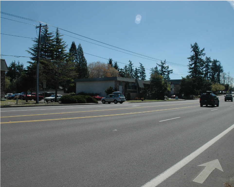
Figure 28. Thinlay placed in 2007; photo taken June 2017
