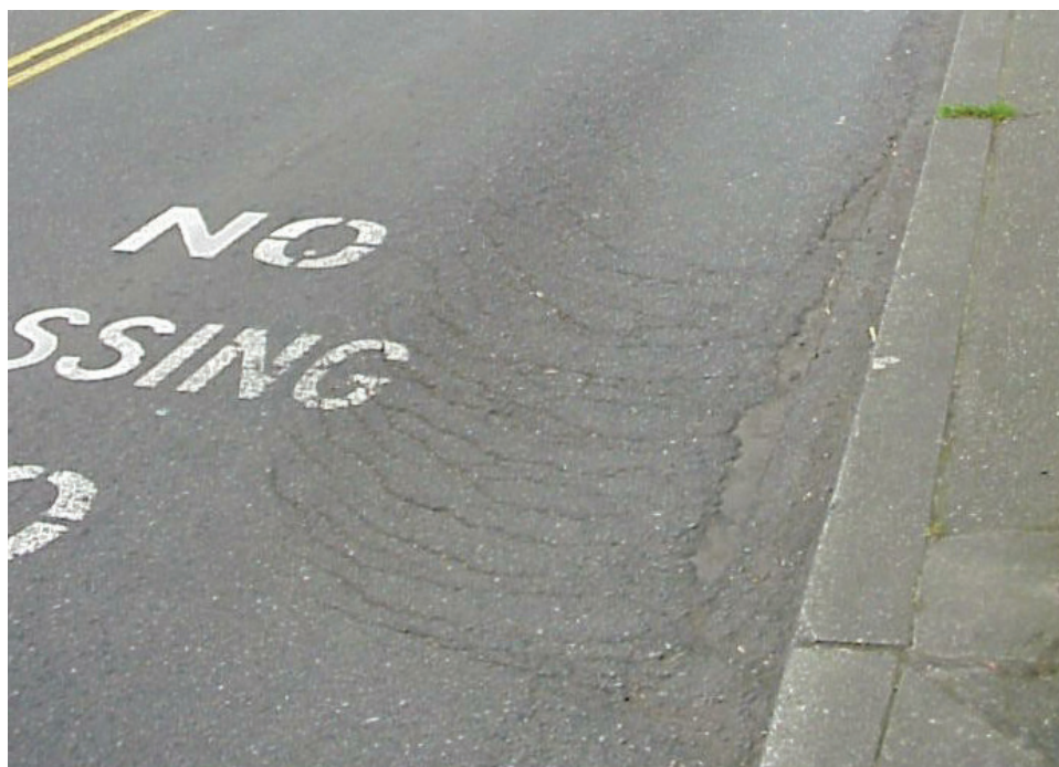
Figure 19. Asphalt pavement slippage
