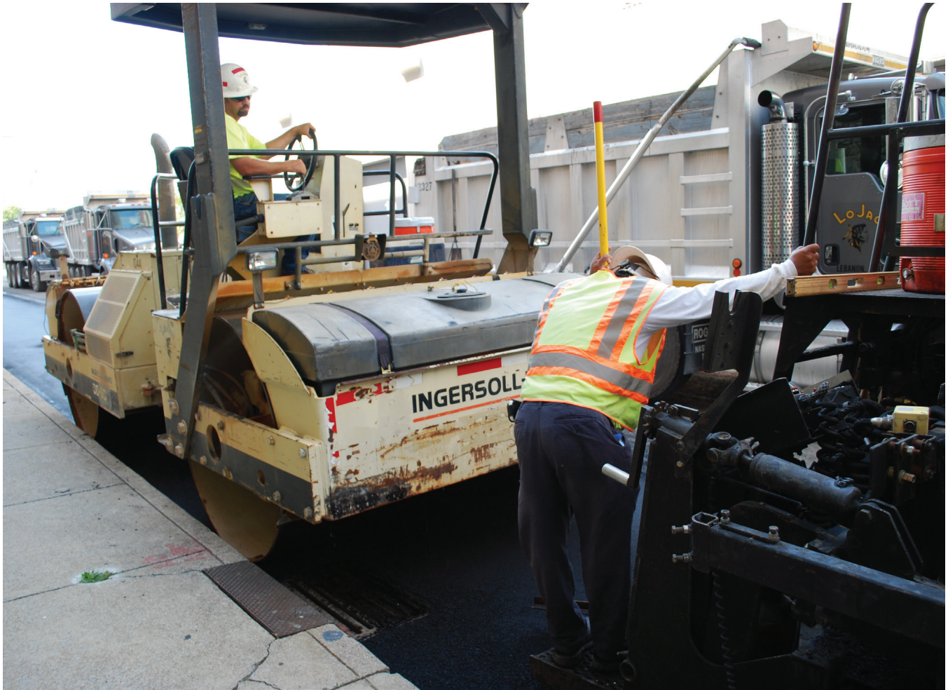
A compactor closely follows the paver on a demonstration Thinlay project in Nashville.
