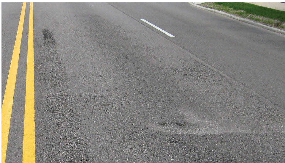
Figure 16. Slight raveling
