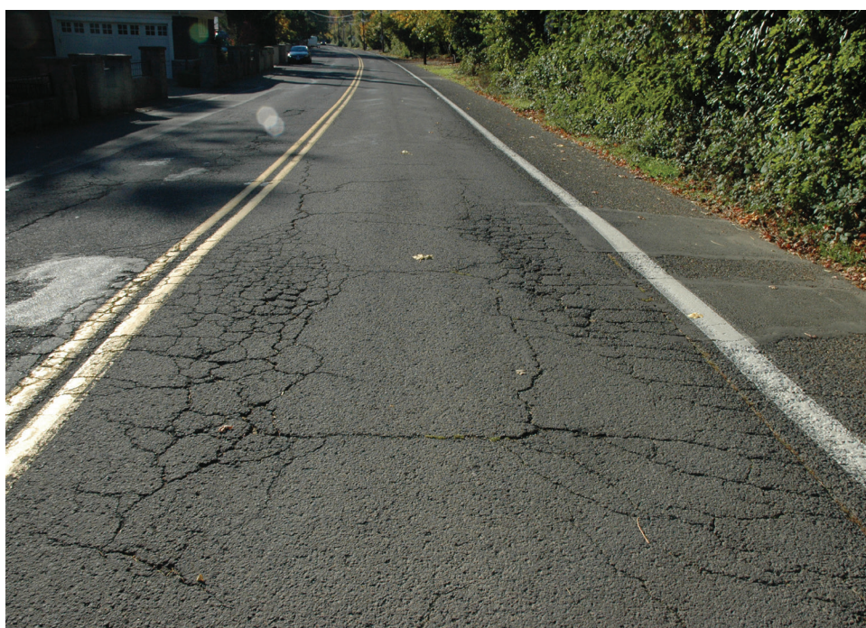
Figure 10. Extensive alligator cracking
