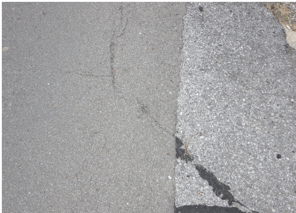
Figure 14. Reflective cracking
