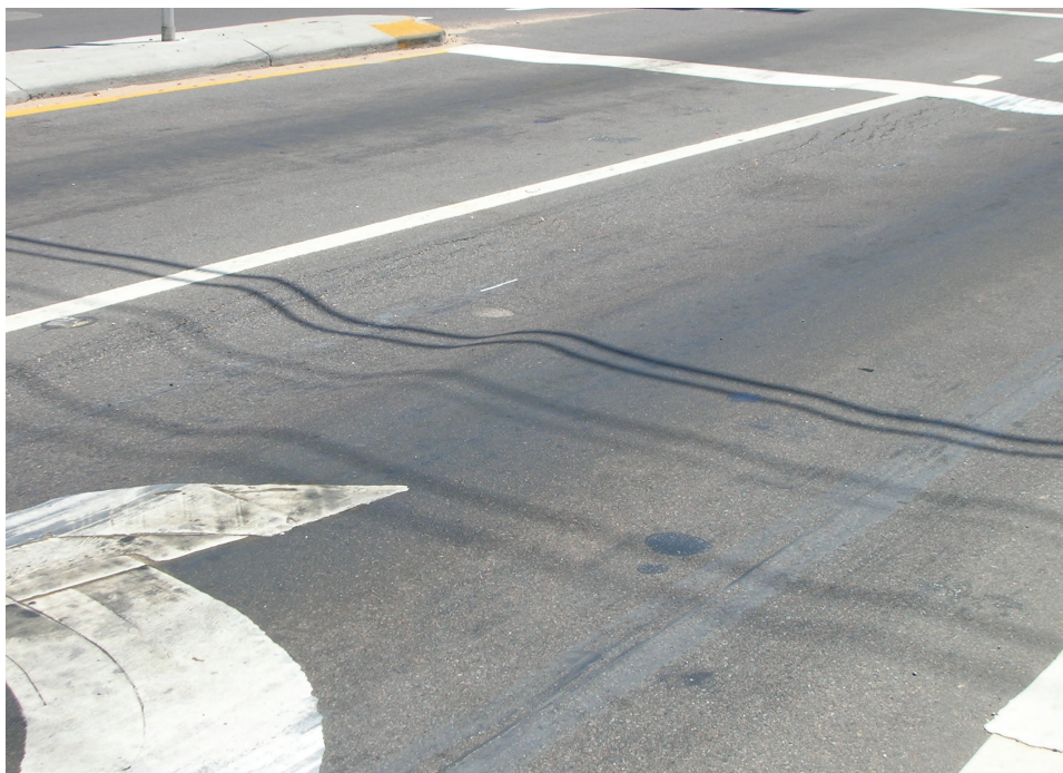
Figure 7. Rut depths exceeding 1 inch
