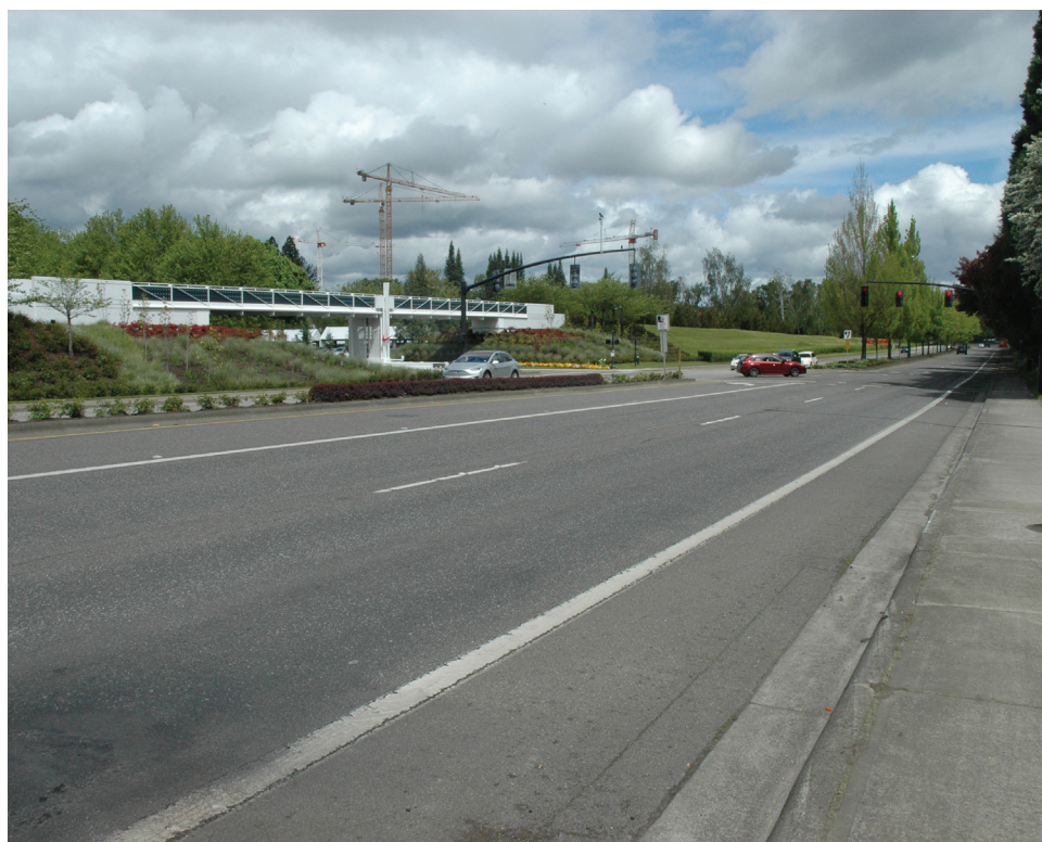
Figure 27. Thinlay placed in 2001; photo taken June 2017
