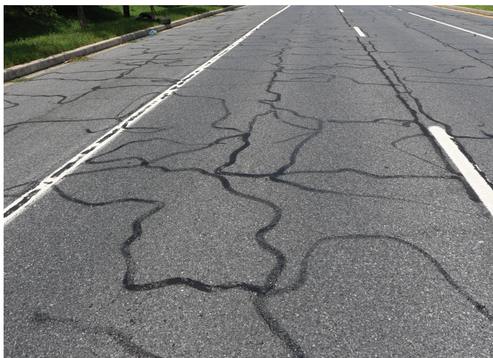
Figure 8. Heavy block cracking with sealed cracks
