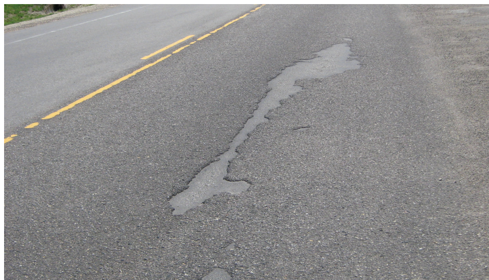
Figure 18. Severe raveling
