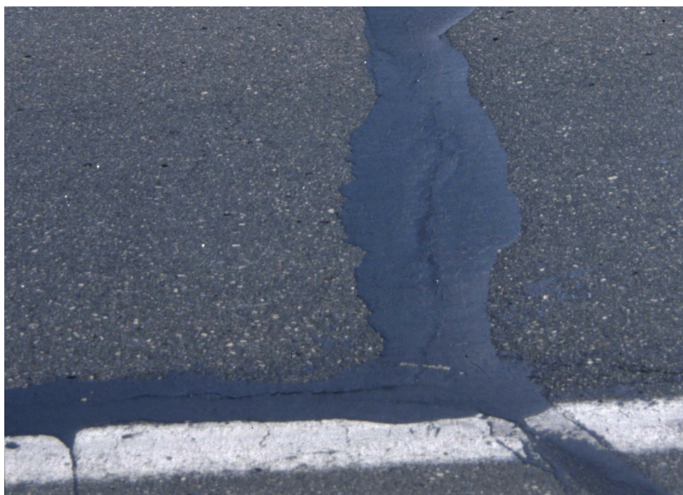
Figure 15. Overbanded crack sealing.
