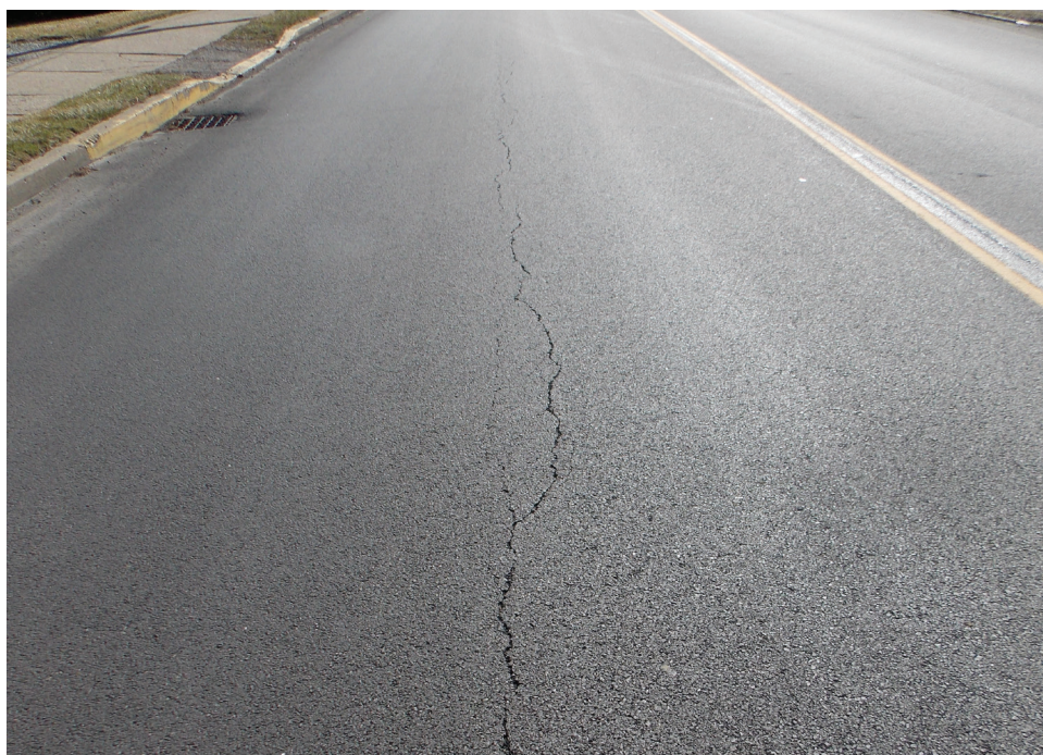
Figure 9. Longitudinal cracking
