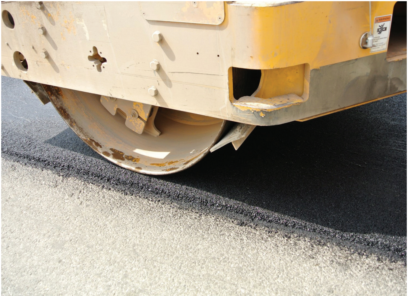
Compaction of a Thinlay mixture
