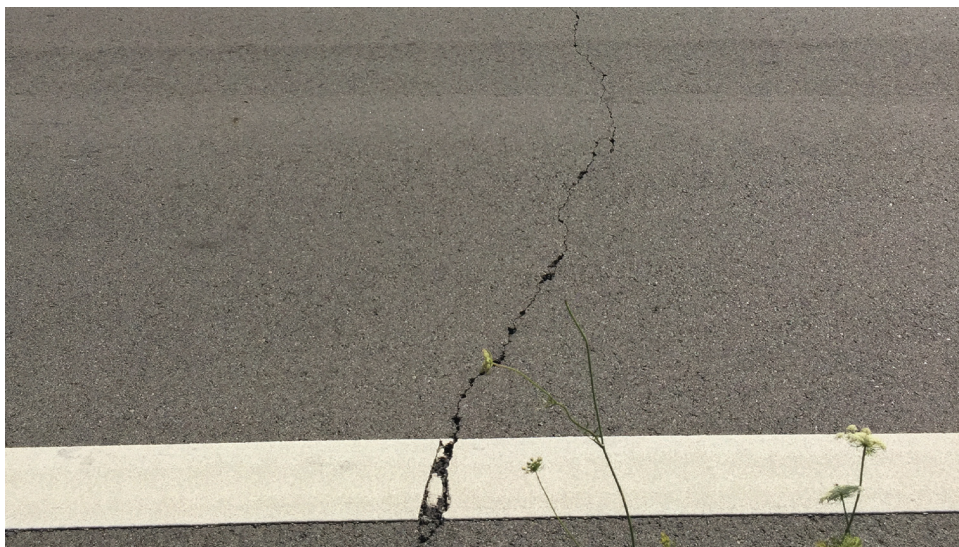
Figure 12. Transverse crack with adjacent deterioration
