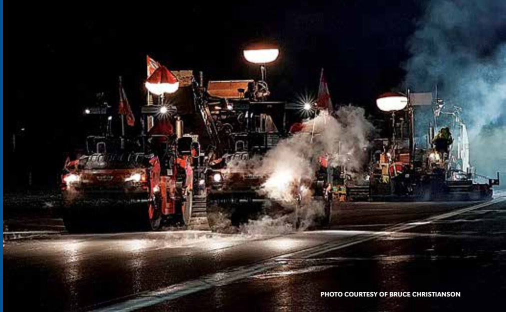
Two IC rollers side-by-side with performing echelon paving.
