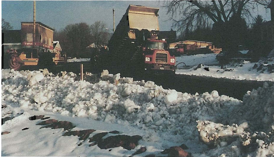
Placing Hot Mix Asphalt (HMA) on the Quincy Hill project, Hancock, Michigan (located on the Upper Peninsula) in November 1991.
