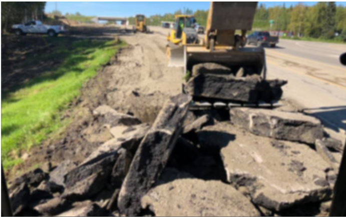
In some places, up to 12 feet of old patched asphalt had to be removed.
