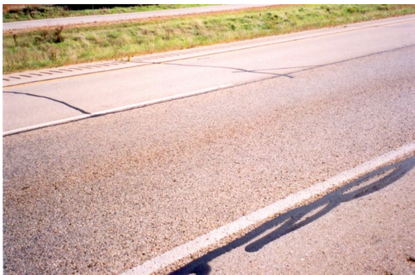
Figure 5.2 Performance of SMA Overlay (near lane) on Concrete Pavement in Wisconsin after 8 Years (Watson and Musselman 2022)
