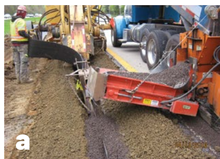
Figure 6.3 Rubblization of JRC: a) Installation of geocomposite edge drain, b) Rubblization of JRC, and c) Compaction of rubblized JRC (Courtesy of NJDOT)
