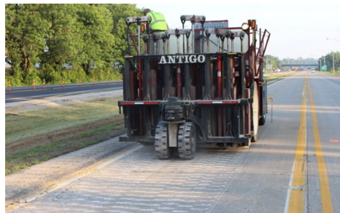
b. Breaking Operation for B&S
