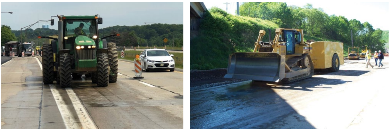
Figure 6.9 Seating JRCF with 50-ton Pneumatic Tire Proof Rollers (Courtesy of PennDOT)
