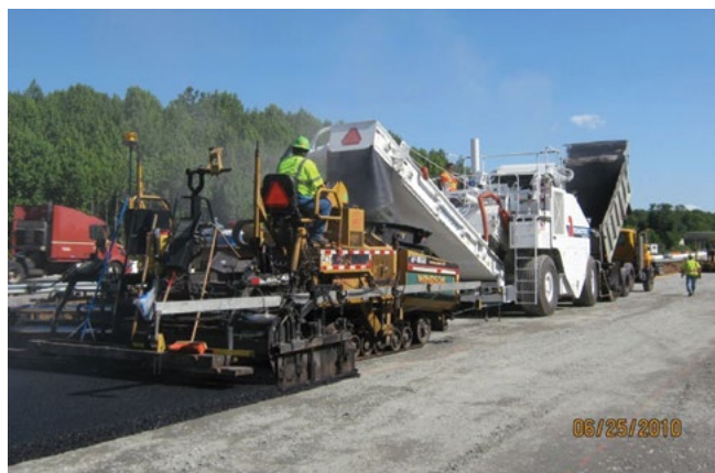
Figure 6.4 Construction of BRBC Layer over Rubblized JRC (Courtesy of NJDOT)
