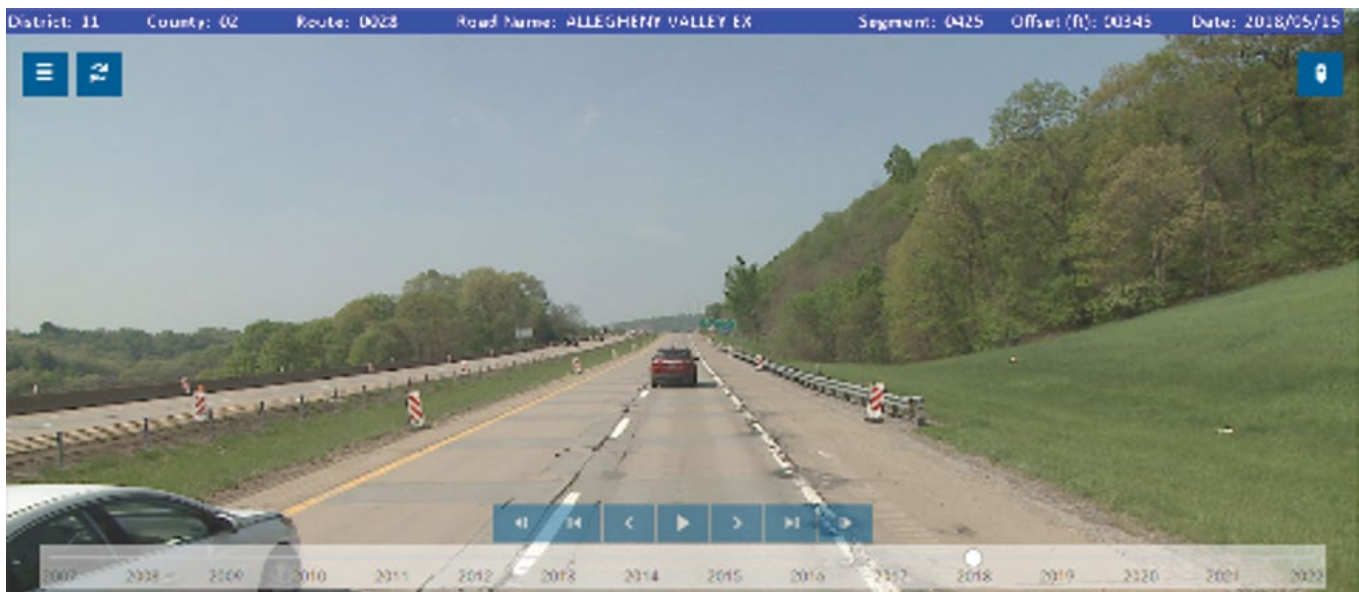
Figure 6.6 Surface Conditions of SR-28, Section A55 in Allegheny County in 2018 Before Rehabilitation (Courtesy of PennDOT)
