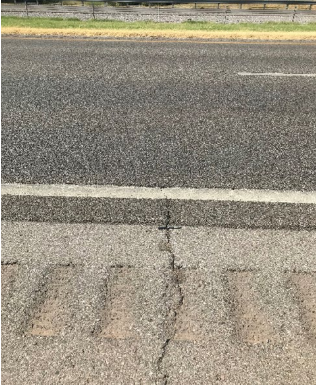
Figure 5.6 HiMA mixture on Oklahoma's I-40 (Vargas-Nordbeck and Musselman 2021)
