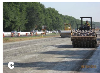
Figure 6.3 Rubblization of JRC: a) Installation of geocomposite edge drain, b) Rubblization of JRC, and c) Compaction of rubblized JRC (Courtesy of NJDOT)
