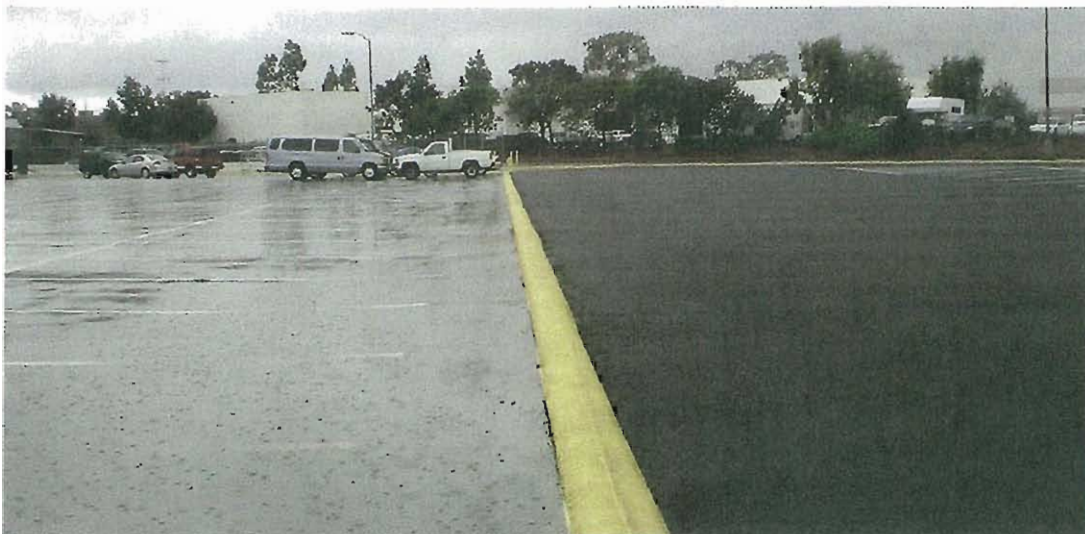
Porous pavement is on the right in this San Diego parking lot.
