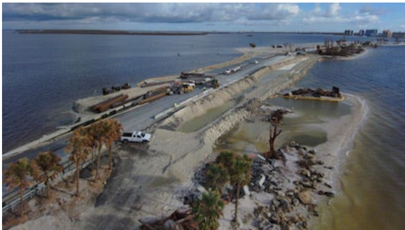
After, Island 1 Breach / Provided by Superior Construction
