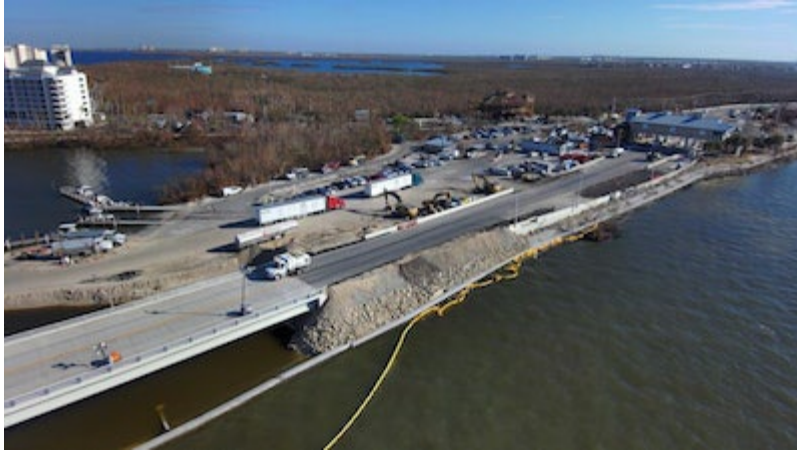
After, Bridge Approach A / Provided by Superior Construction
