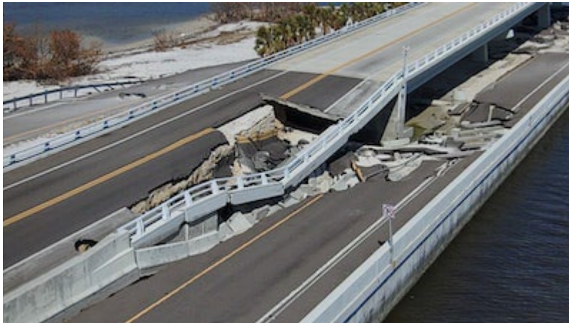
Before, Island Bridge 1 Approach / Provided by Superior Construction
