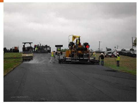
side-by-side and a third in the wide areas of the track for two reasons, one to expedite the laydown operation and second to eliminate a cold longitudinal joint for better compactive effort and joint density. Kirby-Smith Machinery of Oklahoma City brought a Vogele Vision 5200-2i Paver for demo, later purchased by Dunham's. Dunham's also hired the services of Ellsworth Construction to help with the laydown using a Cat AP555E Paver. Where a third paver was needed, a Leeboy 8510 was used.
