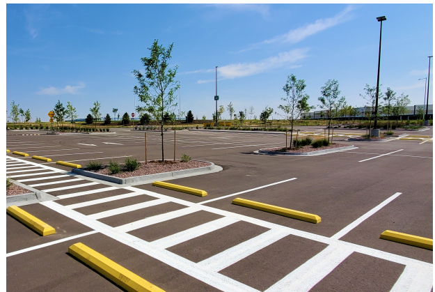
Amazon Fulfillment Center (Colorado Springs), Contractors: Schmidt Construction & Pyramid Construction
