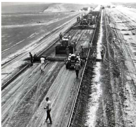
Paving operations near Richardton, N.D., on Interstate 94 in 1967.
