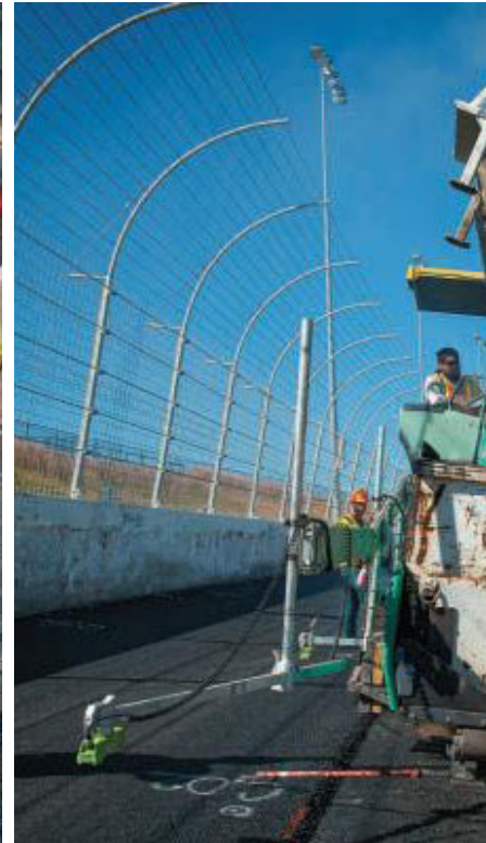
Absent any off-the-shelf equipment options, custom fabrication was required to meet the demands of running heavy paving machinery on a 28-degree incline.
